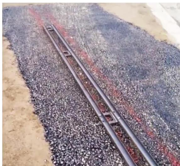
Fig. 7: Preparation of the installation plates by using the drilling template for SMA T2-SMA T4
