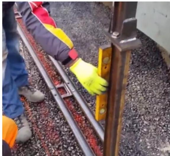
Fig. 10: Check through the spirit level
