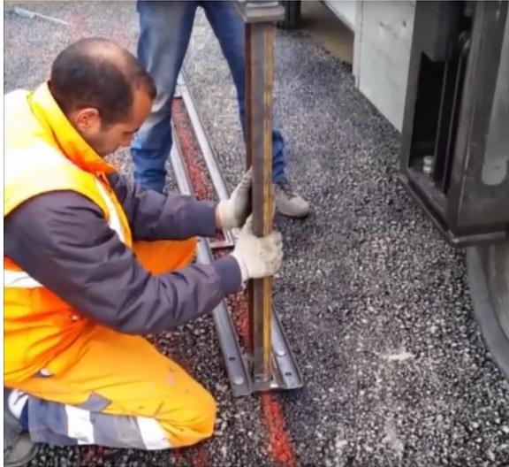
Fig. 8: Insertion of the post type IPE 80 with welded plate.
