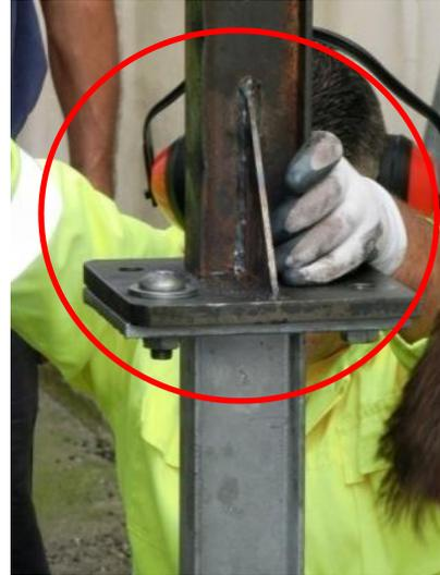
Fig. 9: Tool for the post hammering screwed on the post
